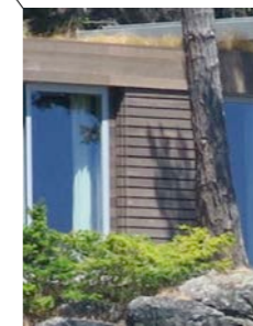
To give a soft warm-to-the-touch feel around the main feature Living room doors and patio area, the underside of the overhang and the wall surrounding the doors will be clad in a Walnut coloured stained wood
