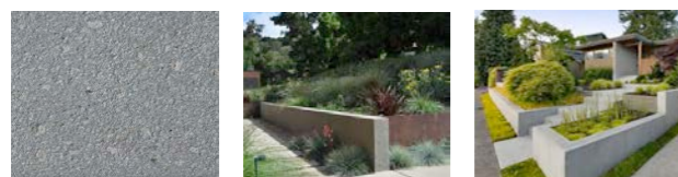
The classically modern design planned for the DVP application house has a modern crisp aesthetic similar to the images shown below: Low, long, lightly sandblasted, and showing a fixed pattern of form tie indentations
