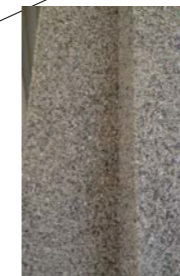
Planned for two areas is the use of a Pebbledash of cream coloured stones with a matching cement coloured stucco. Small sized stones will give a uniform look that is contrasted with the Sand Flat finish areas.
