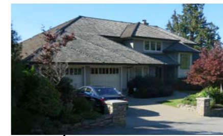
The curving nature of the street brings the road right to the edge of the property across the street, whereas with 6236 - the property in question has a 16 ft wide Boulevard in front - the opposite condition.
