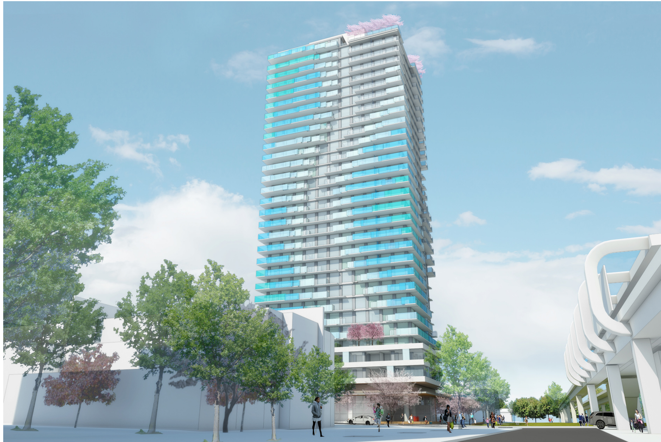
View from Vanness Avenue Looking East
