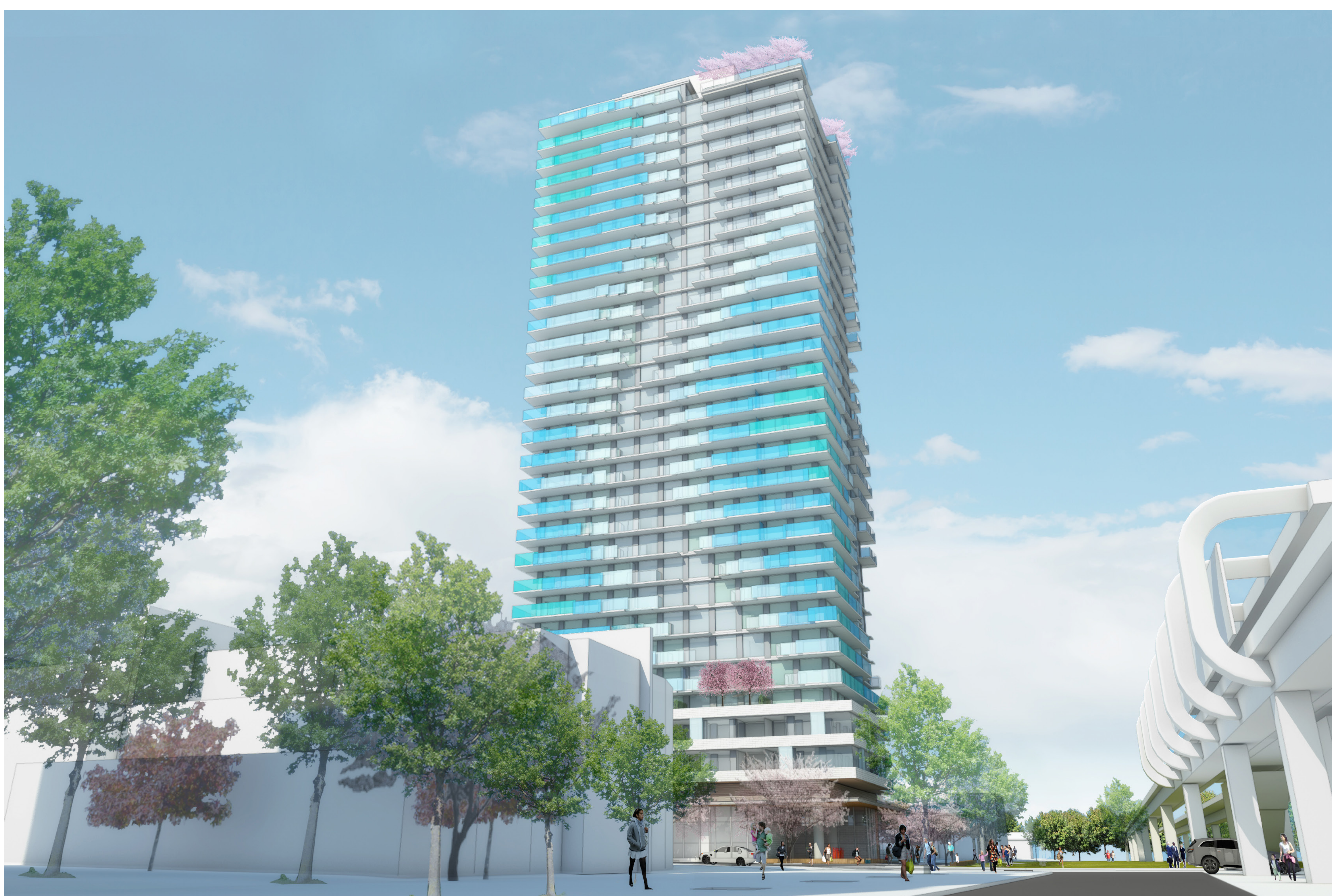
View from Vanness Avenue Looking East
