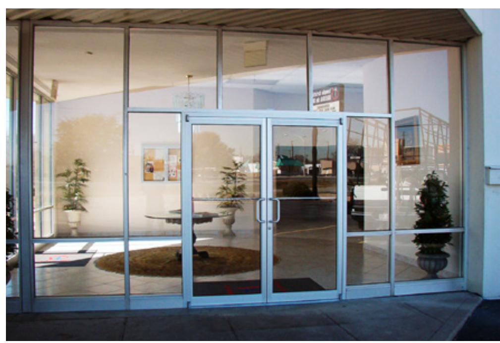
① Clear Glazing in Aluminum Frames
