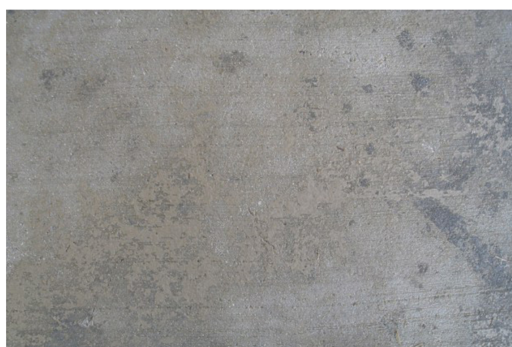
⑦ Architectural Concrete
